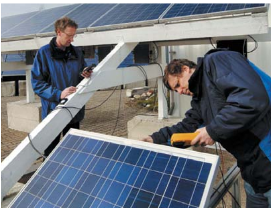
Installation of Photon Lab's outdoor module test. Photo: photon-pictures.com
